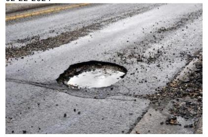
The Town will fill potholes as weather allows, but the freezing and thaw cycle of Colorado winters is not ideal for patching. The Public Works department will fill some priority potholes on particularly warm days.
